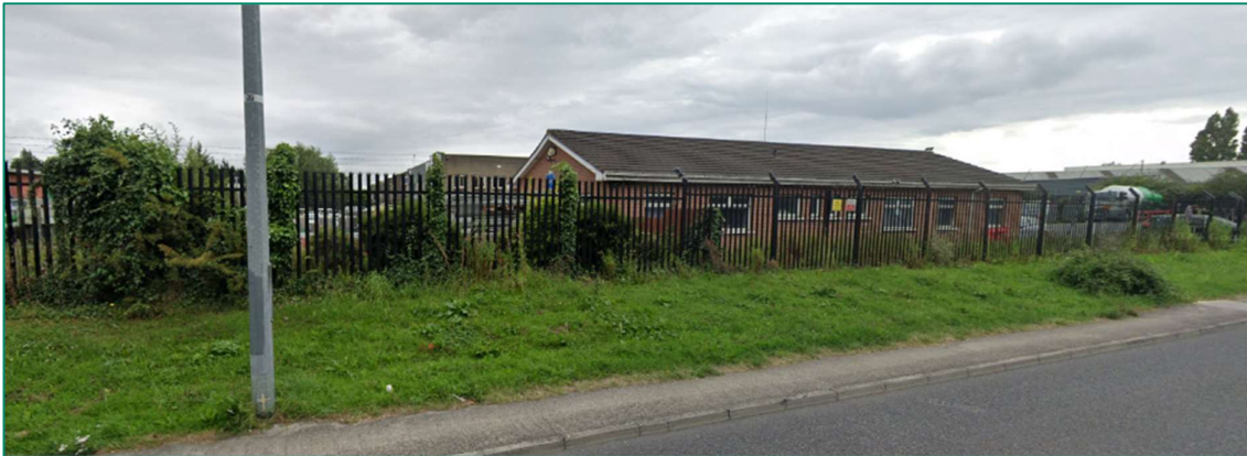
Figure 2.1.5: Existing boundary fence to Air Products Ireland Limited (Image source: Google)
