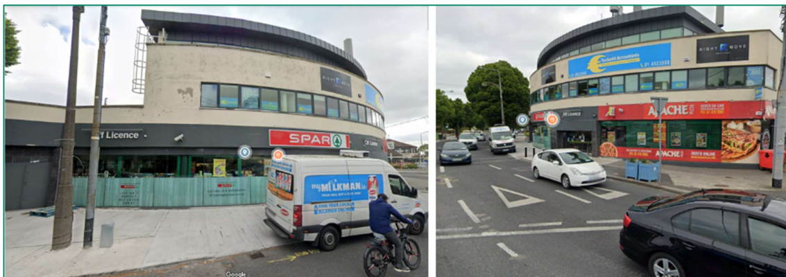
Figure 2.11.5: Existing footway outside Spar and Apache Pizza; no existing on-street parking (Image source: Google)
