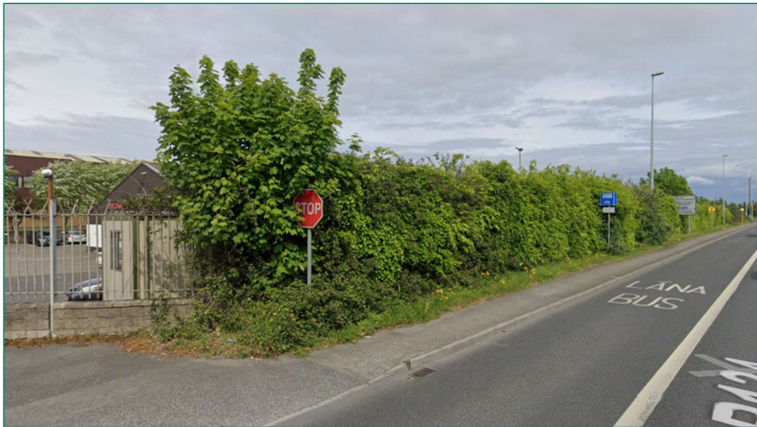
Figure 2.22.6 Existing boundary to Toyota Motor Group east of the central gate (Image source: Google)
